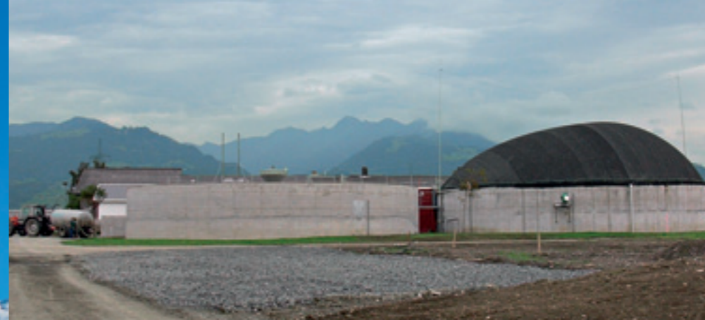
Biogasanlage Gstach in Rankweil.
